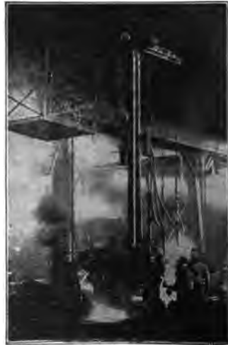
FIG. 188.—Ramming Molds—the First Step in Molding a Cast Iron Pipe. A large cast iron flask is placed in a pit and a pattern is placed in the flask. Sand is then filled in around the flask and rammed down hard. In this case, the rammers are driven by compressed air and are suspended by a stationary overhead crane. The pattern is then drawn and the mold is ready for the core.
